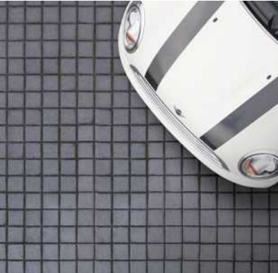
Firth precast concrete modular paving ('Holland' modules) to key pedestrian entry points into the site (flush with adjacent concrete surface).
