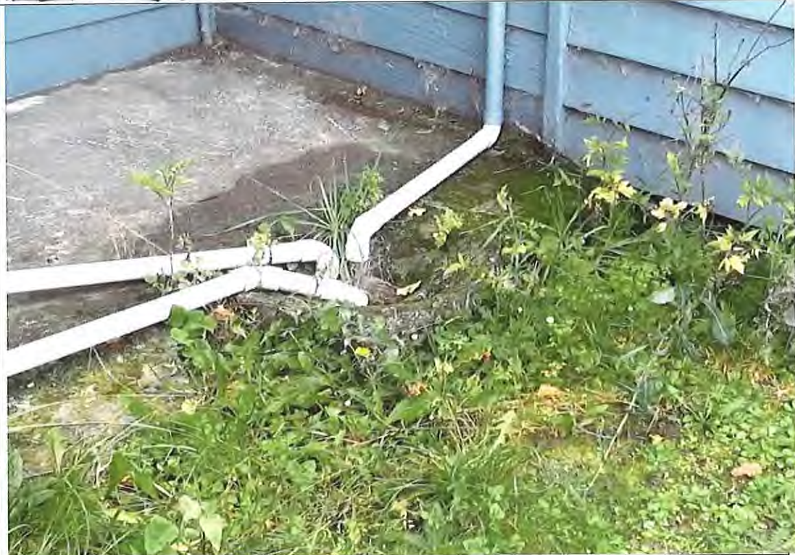
Problem: Low Gully trap allows water ingress into sewer pipe.
