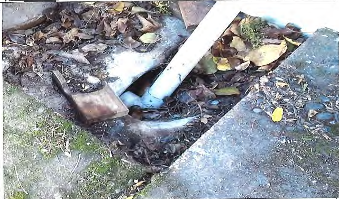
Problem: Low Gully trap allows water ingress into sewer pipe.
