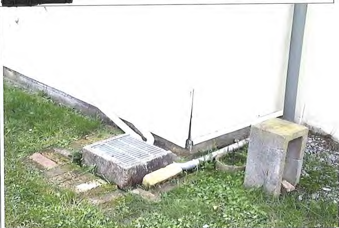
Problem: Gully trap will allow ingress of surface water and the down take pipe water.
