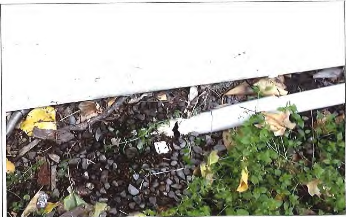
Problem ( [REDACTED] ): Damaged Sewer Pipe allow ingress of surface.
