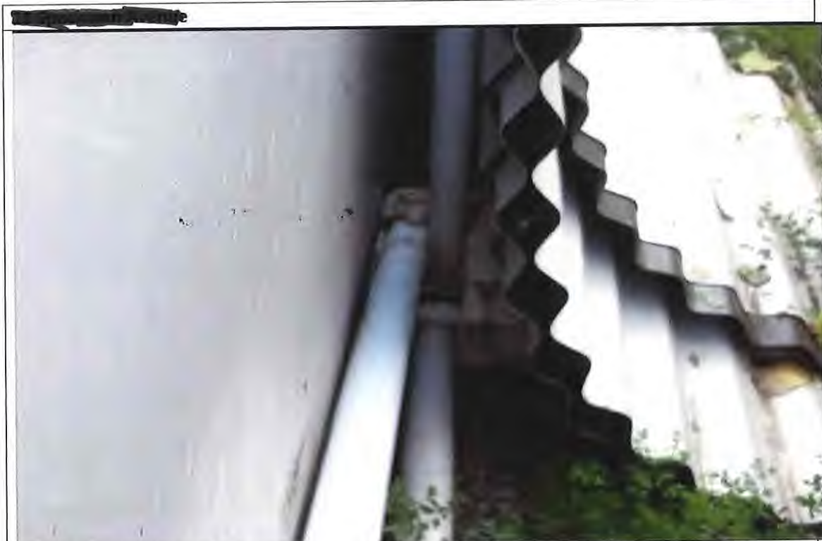
Roof down pipe flows into Gully trap.
