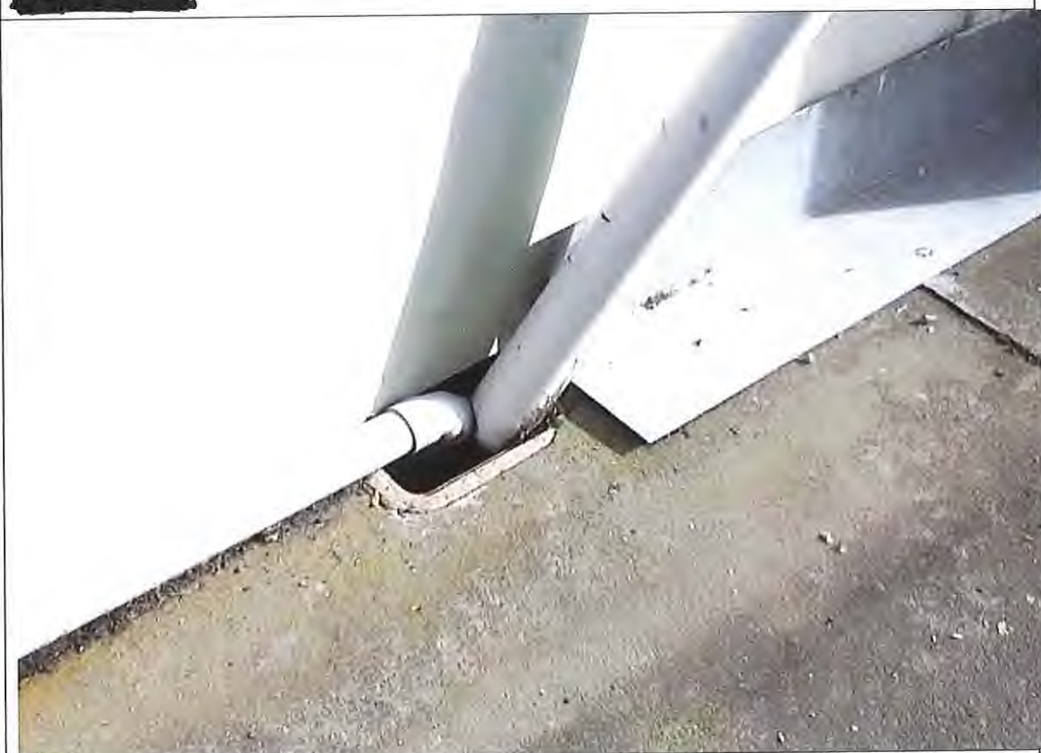
Problem: Low Gully trap allows water ingress into sewer pipe.
