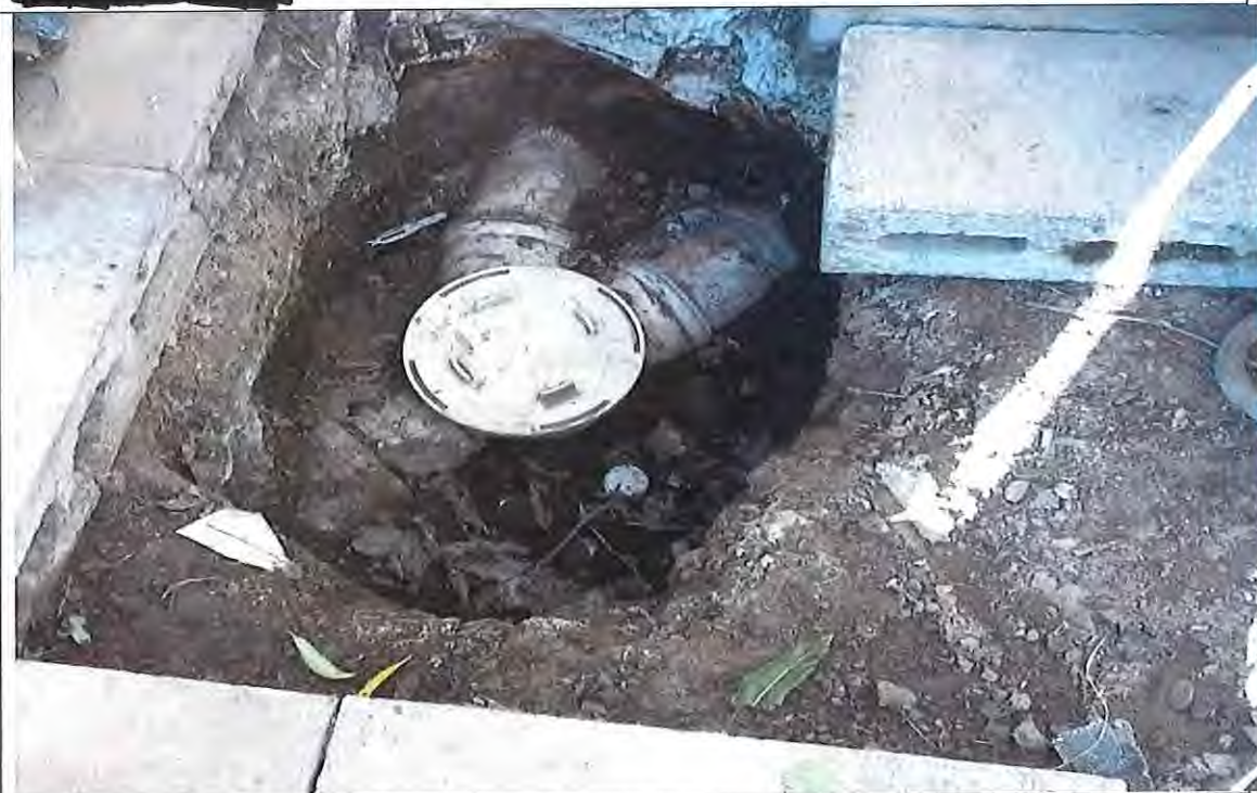
Problem: Non-compliant Gully trap, may allow water ingress into sewer pipe
