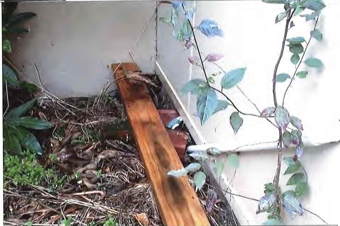
Problem: Low Gully trap allows water ingress into sewer pipe.
