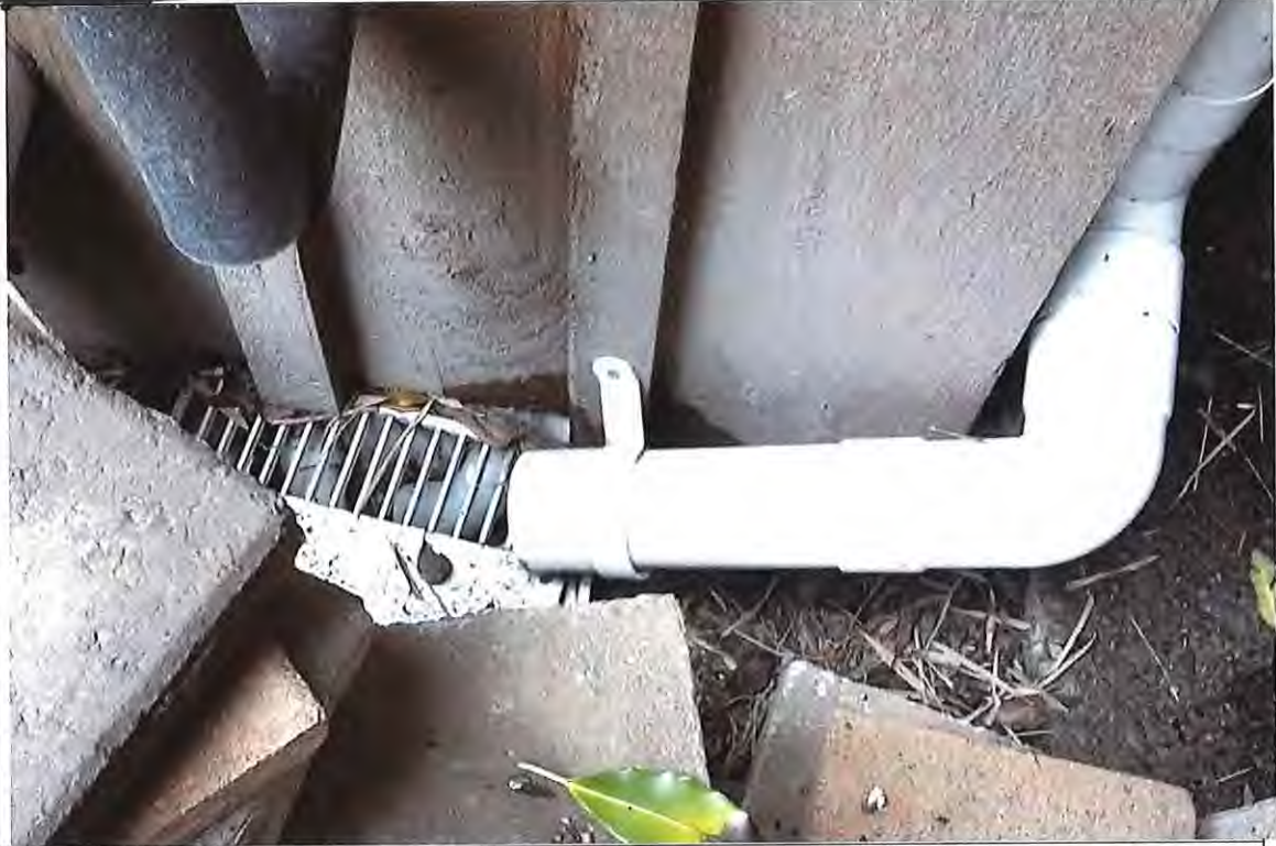
Problem: Roof down take pipe connected to GT
