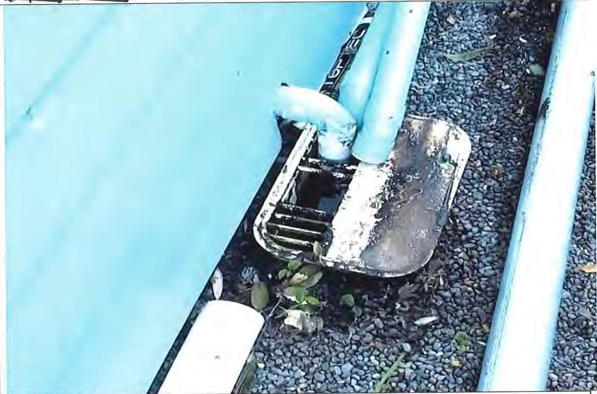
Problem: Roof water down take pipe close to GT.
