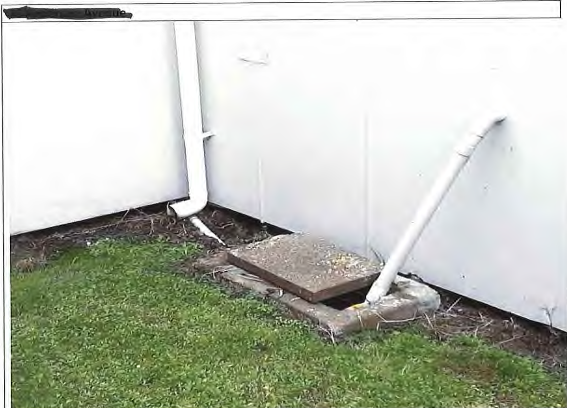
Problem: Low Gully trap that may allow water ingress. Roof down take pipe close to GT
