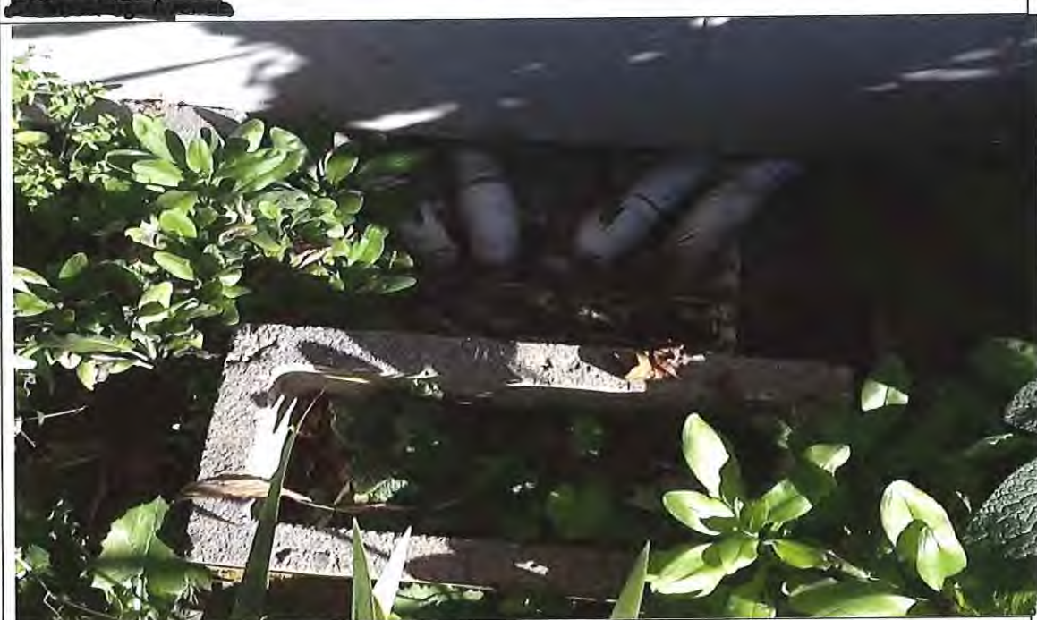
Problem: Low Gully trap allows water ingress into sewer pipe.
