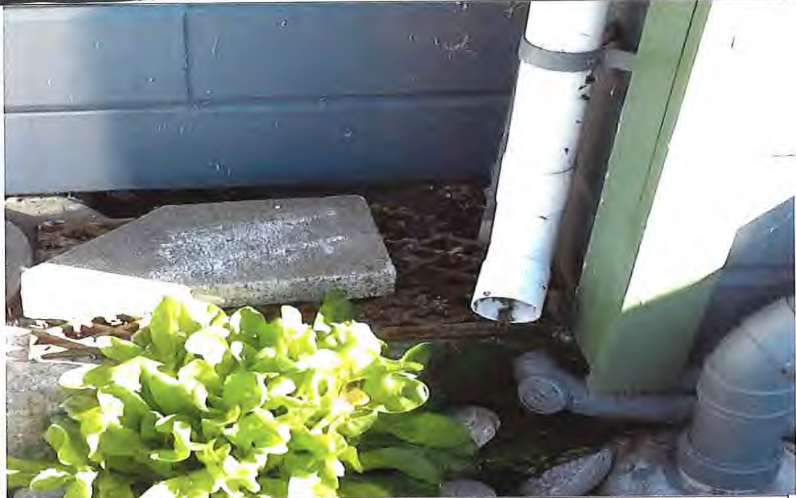
Problem: Roof down take pipe connected too close to GT.
