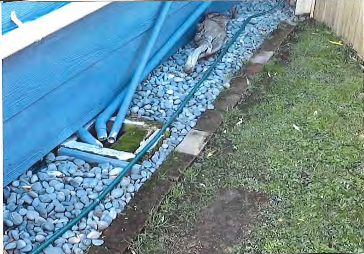
Problem: Low and Damaged Gully trap allows water ingress into sewer pipe.
