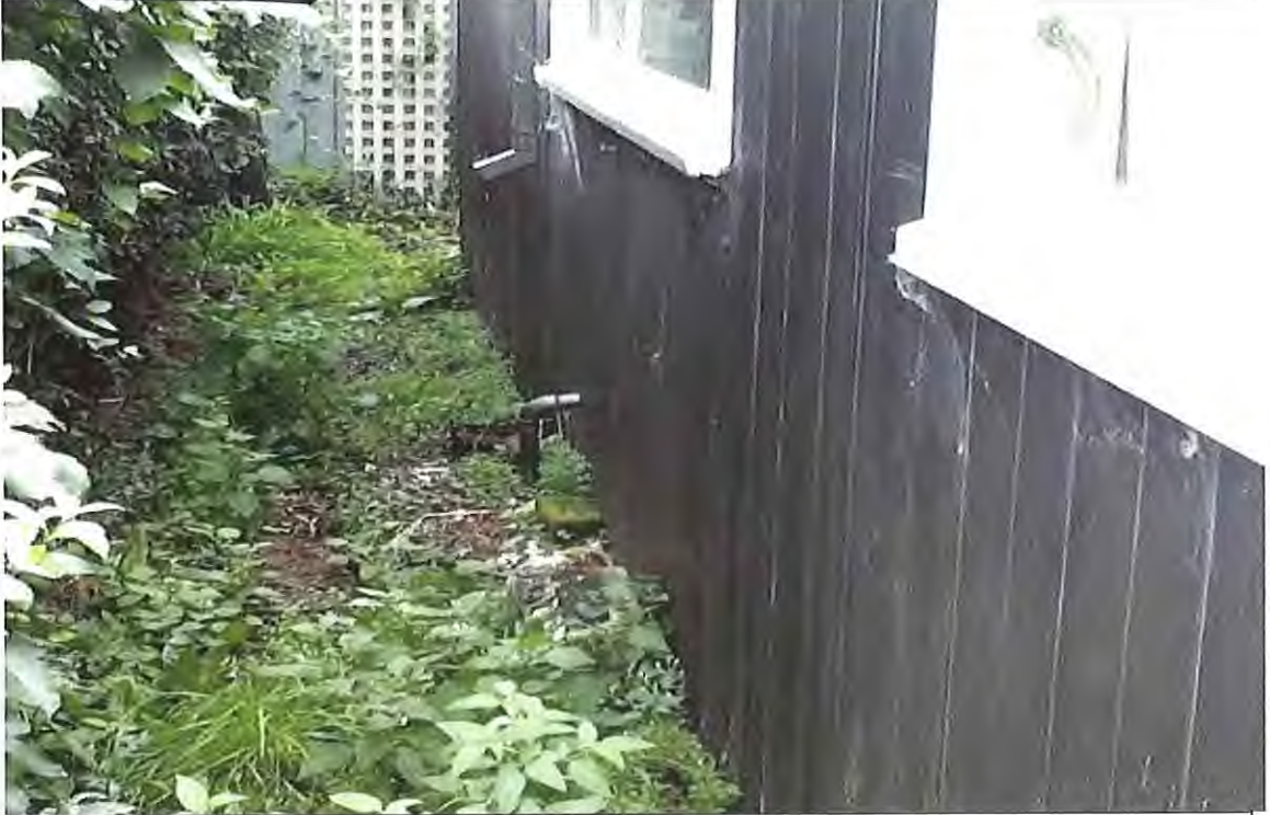
Problem: Low Gully trap allows water ingress into sewer pipe.
