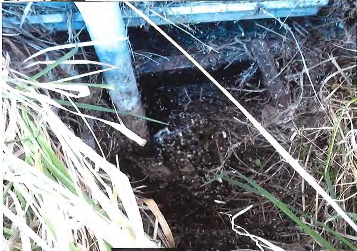
Problem: Damaged Gully trap allows water ingress into sewer pipe
