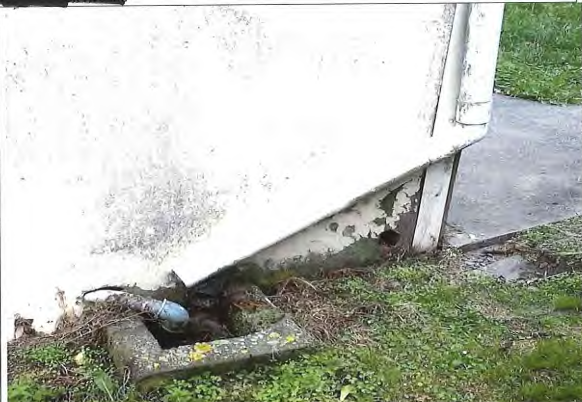
Problem: Low Gully trap allows water ingress into sewer pipe. Roof down take pipe flows into GT
