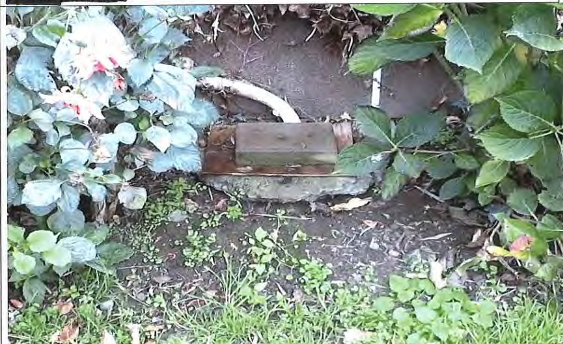
Problem: Low Gully trap allows water ingress. GT needs repair
