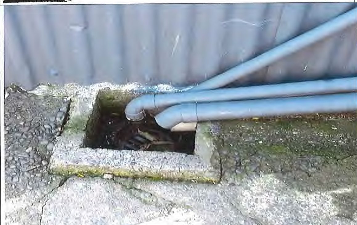
Problem: Low Gully trap allows water ingress. Appears to have roof down take pipe connected
