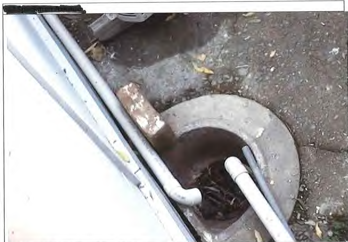
Problem: Gully traps is flushed with the ground and will allow ingress of surface water.
