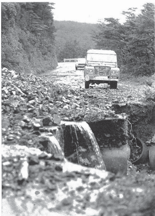
Figure 21: Flood and debris flow damage to SH73 at Snow Creek, 3 December 1979.
