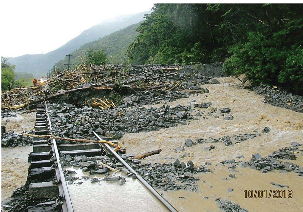
Figure 24: Debris flow in rail formation north of Halpin Creek.
