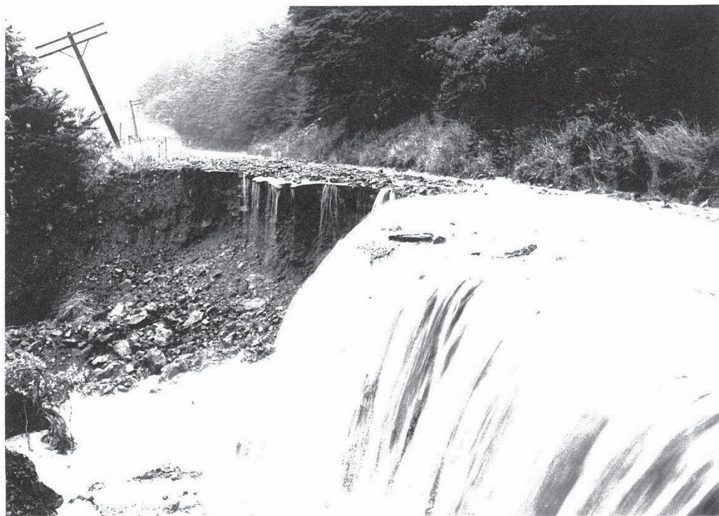
Figure 22: Erosion of road formation due to flooding near Snow Creek, 3 December 1979.
