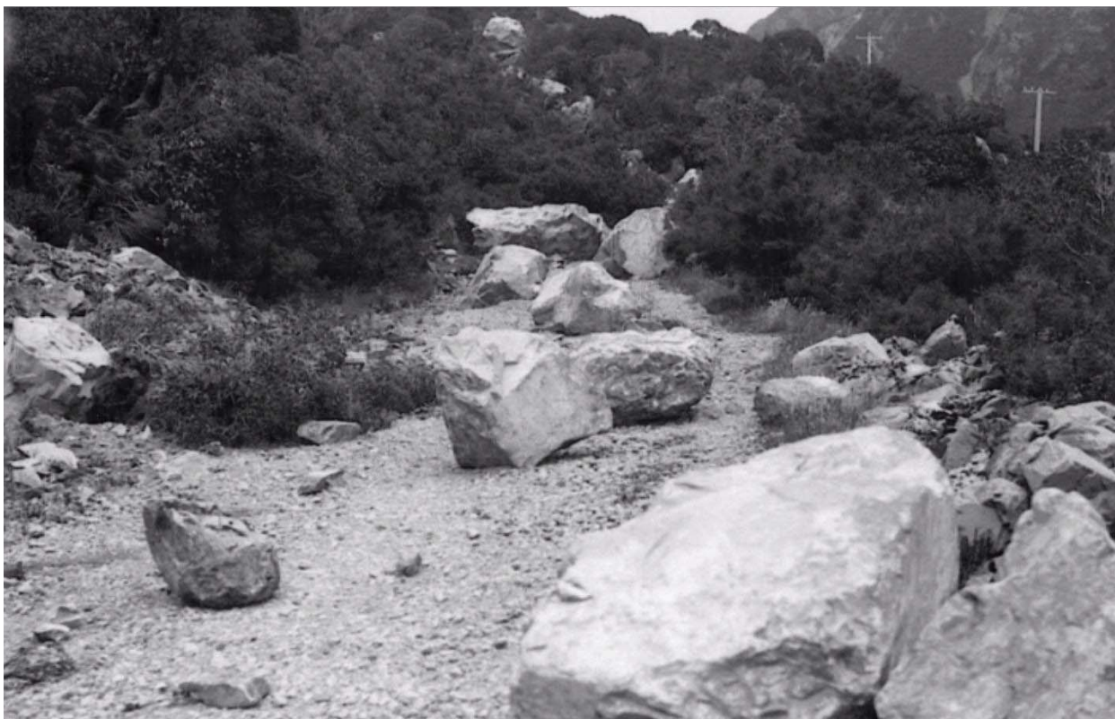
Figure 4: Rockfall onto SH73 at the Zig Zag (Otira side of Arthur's Pass) as a result of the 1929 Arthur's Pass earthquake.
