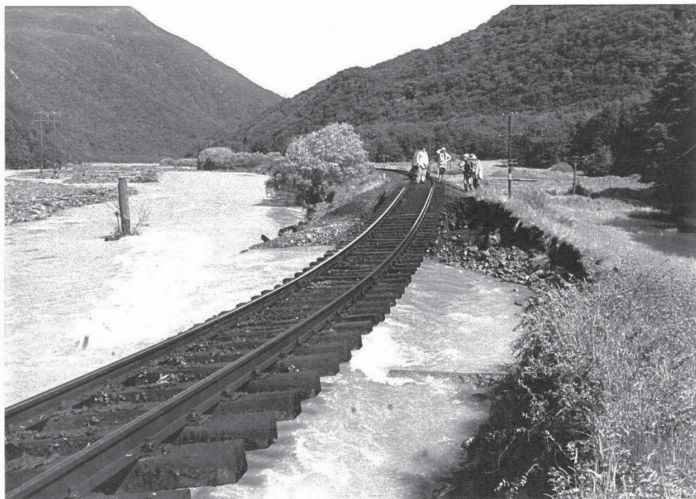
Figure 27: Erosion of rail formation by Bealey River near Halpin Creek.
