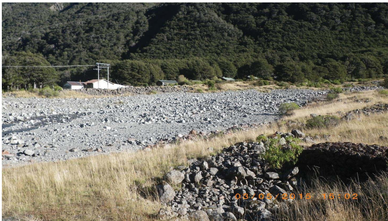
Figure 20: Channel of Rough Creek showing flood protection banks.
