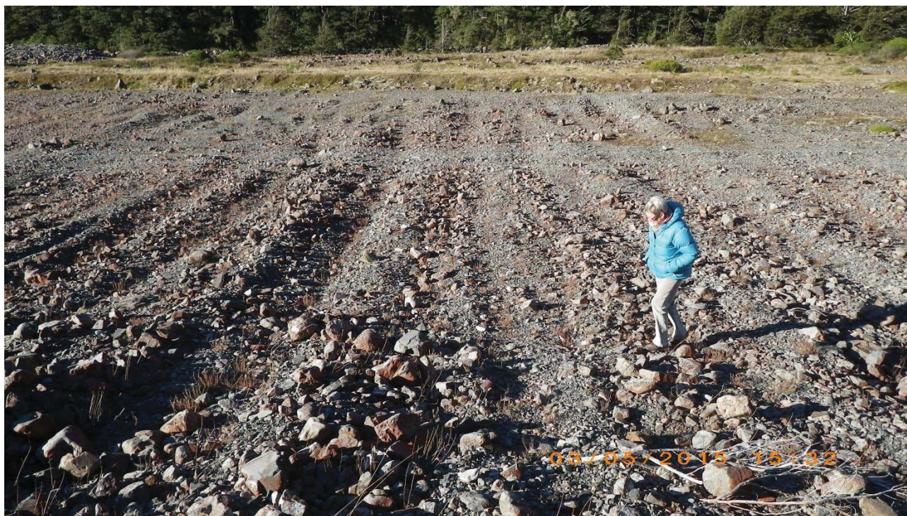
Figure 16: Channel contouring in the flood plain of the Bealey River.
