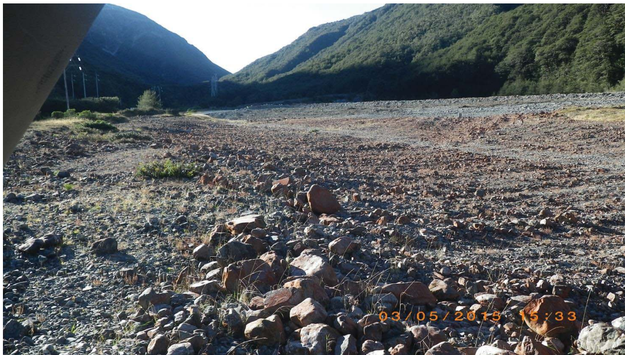
Figure 17: Contoured flood channel for the Bealey River.
