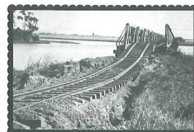
Fig. 9 – Collapse of rail embankment (1931 Napier Earthquake).
