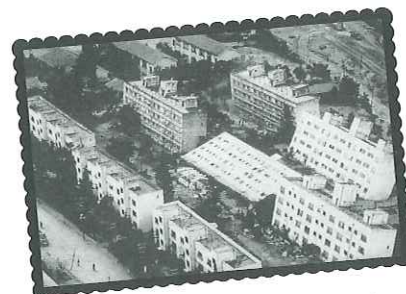
Fig. 7 – Tilting and toppling of buildings (1964 Niigata Earthquake, Japan).
