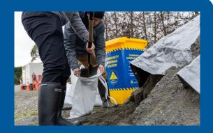
In an emergency, sandbags can be used to block doorways and other openings into properties to keep water out for short periods. Water does seep through sandbags, even when well-stacked and trodden into place. This can be improved by using them in conjunction with plastic sheeting.
