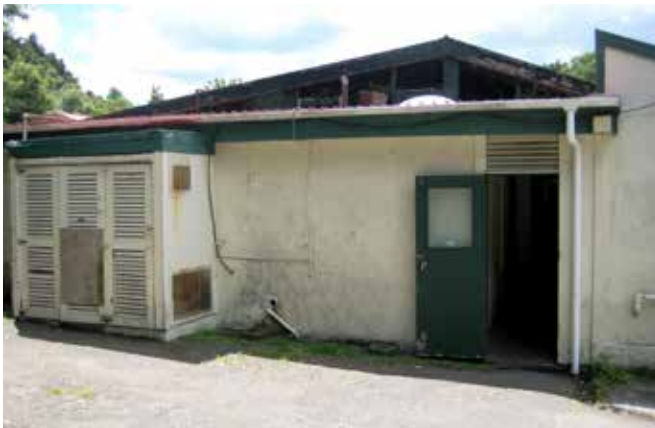
Example of unlit rear of a bar
