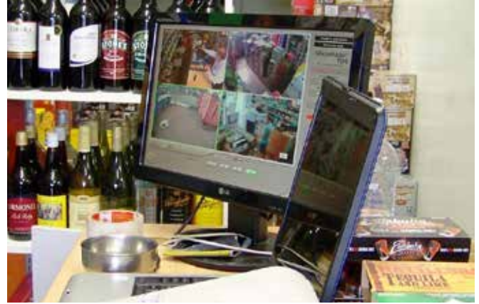
Example of CCTV monitor
