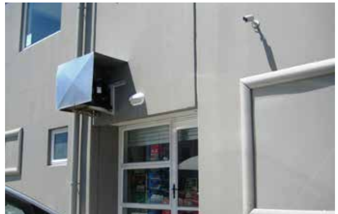
Example of CCTV at rear of premises
