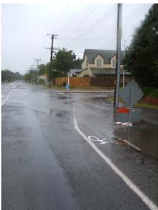
Figure 6 Ponding on Boundary Road corner Birchs Road
