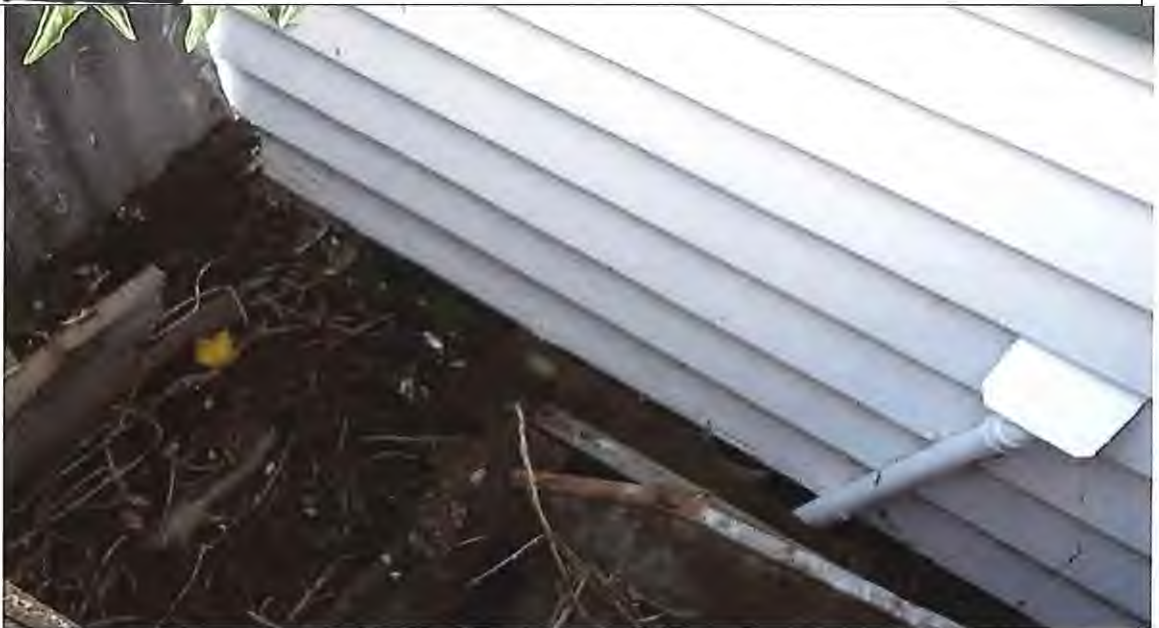
Problem: Low Gully trap allows water ingress into sewer pipe.
