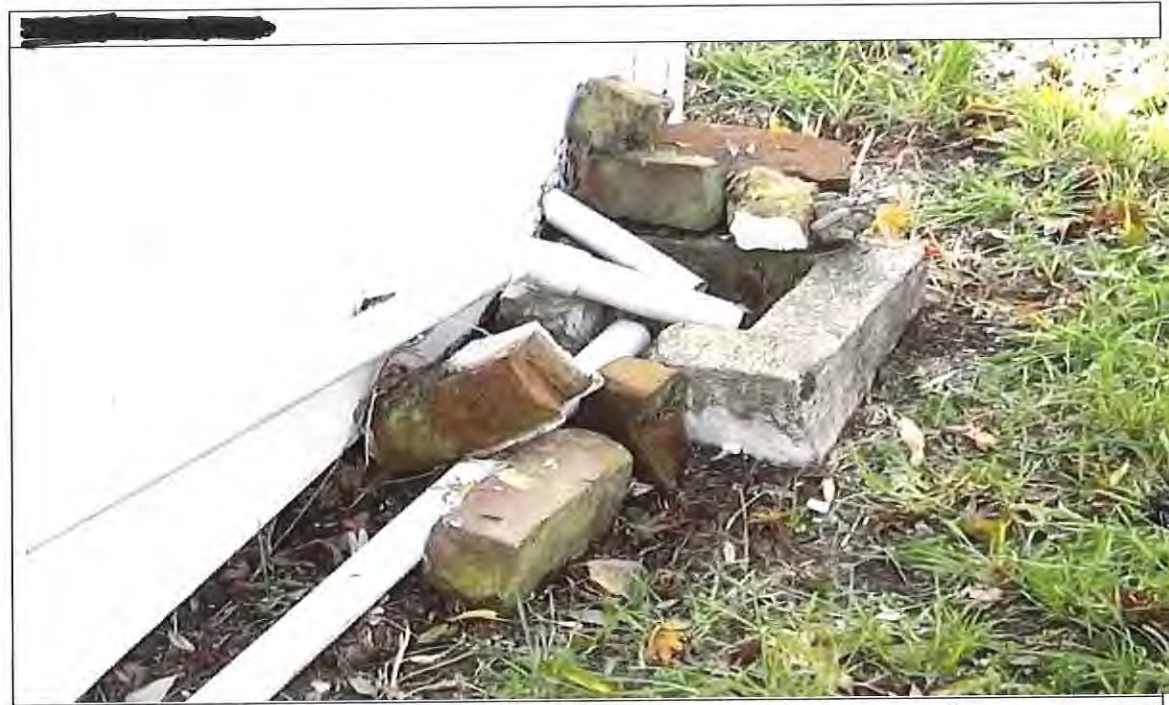
Problem: Gully trap is damaged and can allow storm water to ingress into sewer line.
