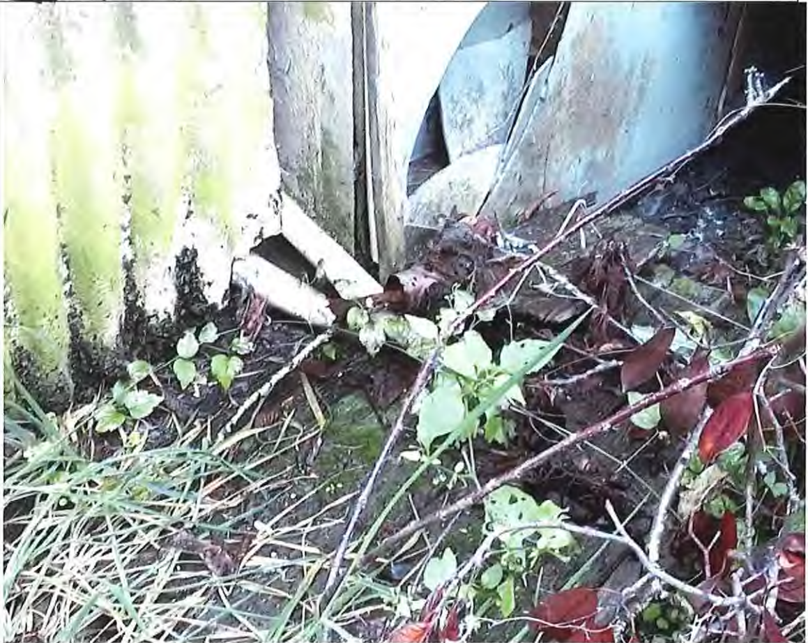
Problem: Low Gully trap allows water ingress into sewer pipe.
