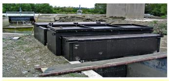
This modern fish screen at the Paparua Intake is a typical example of what may be required at the three Ellesmere water race intakes. The cost of these is around \$160,000 per intake including a fish screen & telemetry.
