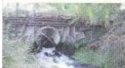
A badly installed culvert – placed too high above the stream bed to allow fish passage.
