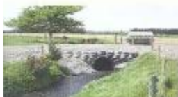
A well-installed culvert
