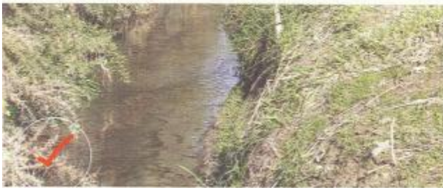
A race that has been cleaned with spoil positioned neatly on the water race bank
