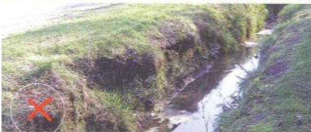
Cutting into the edge of the race bank is not permitted
