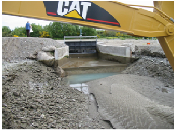
Digger is use to remove silt in weir
