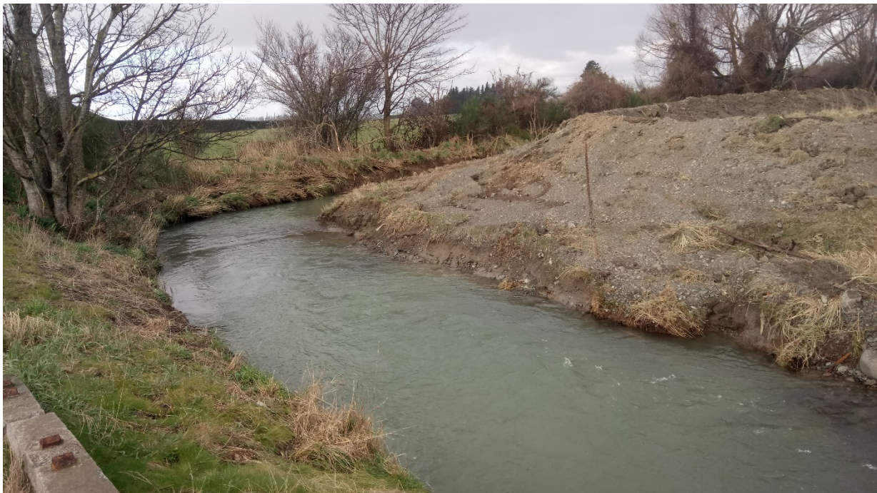
(Picture 5 - Gravel Removed below Railway Yard – Post Flood 2017)
