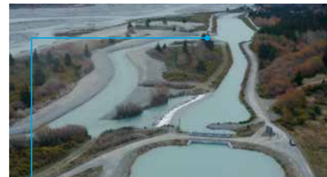
The labyrinth weir's angled or zigzagging weir panels provide a greater weir length within the channel and therefore greater spill capacity than a straight weir.
