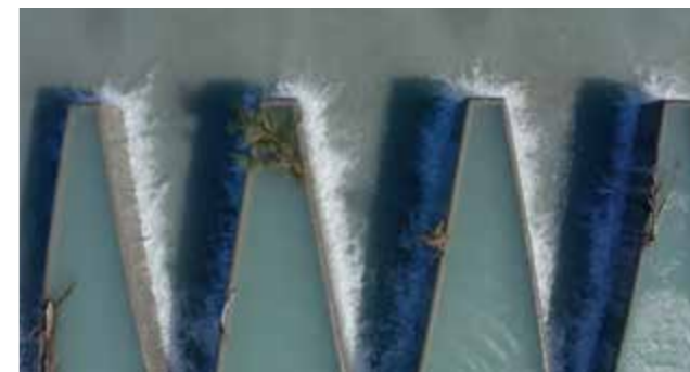
The labyrinth weir's angled or zigzagging weir panels provide a greater weir length within the channel and therefore greater spill capacity than a straight weir.
