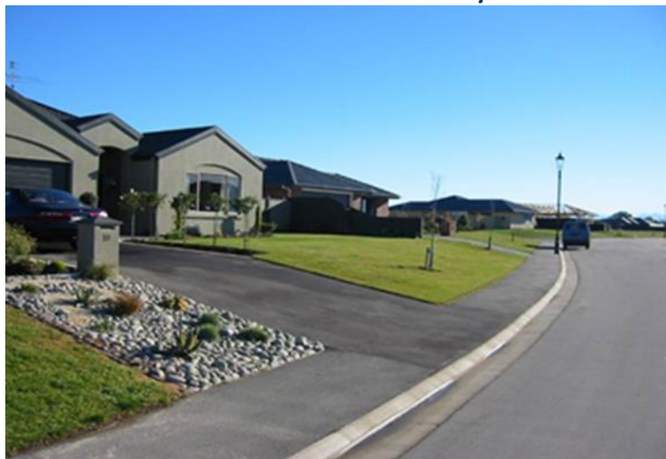
Figure 9.1.2: Low Profile Kerb and Channel and Entranceway
