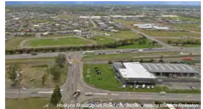
Hoskyns Road/Jones Road intersection, looking towards Rolleston
