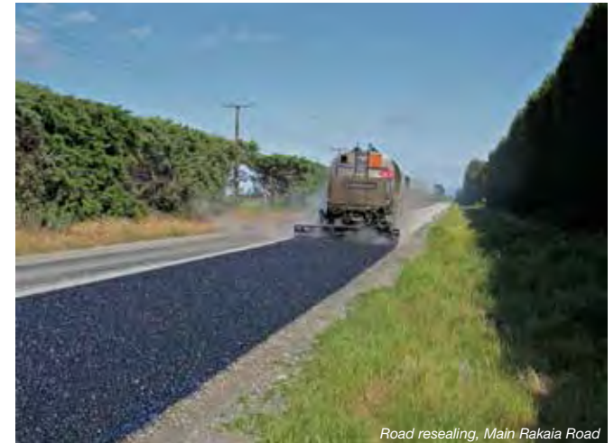
Road resealing, Main Rakaia Road
