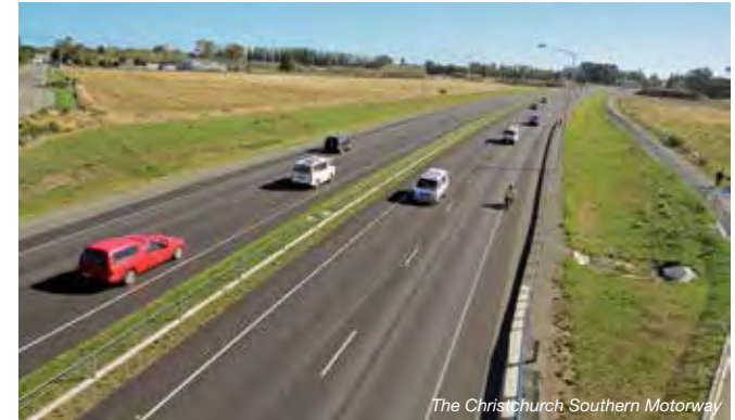
The Christchurch Southern Motorway
