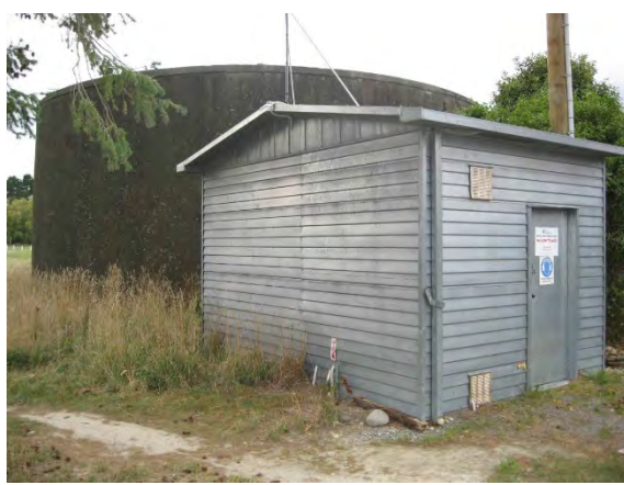
Photo 2: Reservoir and Pump Shed
