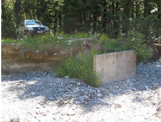
Photo 1: Northern End of Intake Structure
