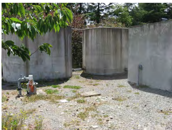
Photo 1: Wellhead, Tanks and Pump Shed
