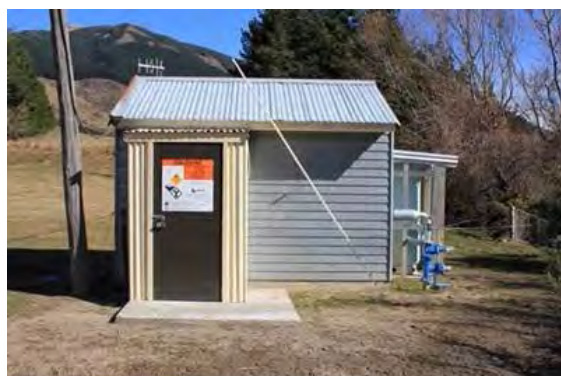
Photo 1: Dalethorpe Treatment Building
