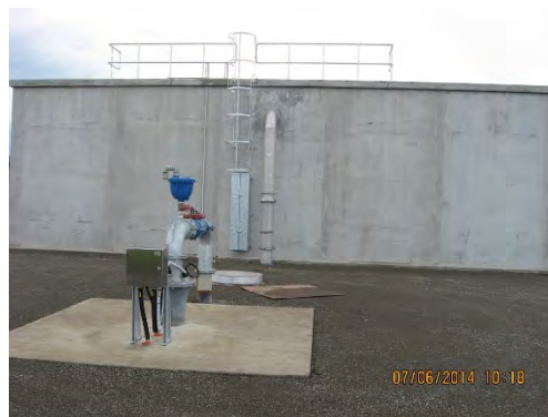
Photo 2: SH73 Bore No 2, Reservoir
