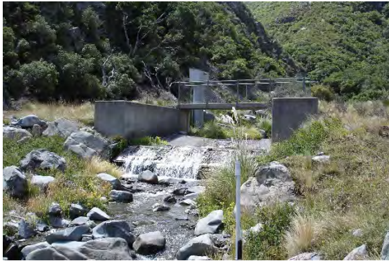
Photo 1: Dry Acheron weir and intake structure
