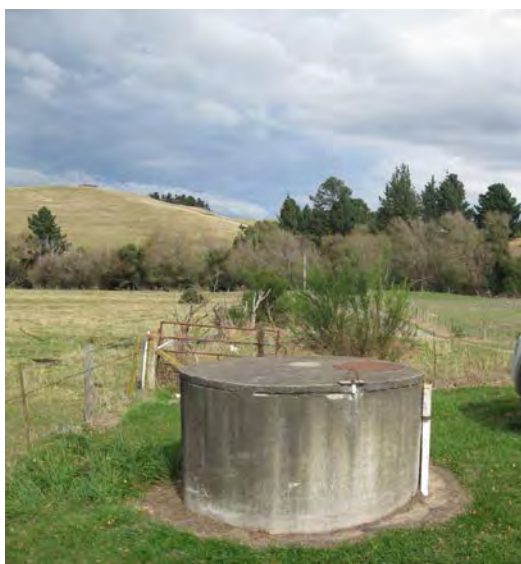
Photo 1: Well No. 2 (typical of both wells) with Reservoir on hill in background (Well No. 1 further along road)
