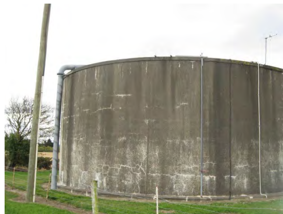
Photo 4: Kimberley Road Reservoir
