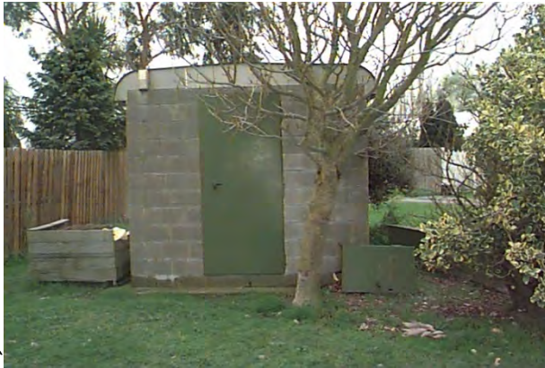
Photo 1: Taiaroa Street Control Building
