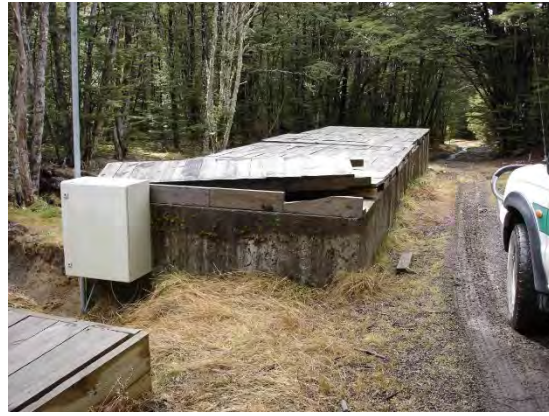
Photo 2: Silt Trap (lid been replaced)
