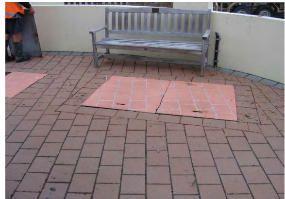
Photo 2: High Street Well head (below covers)
