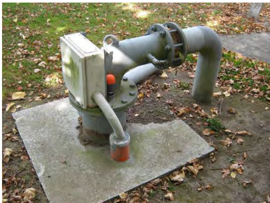
Photo 3: West Belt bore headworks
