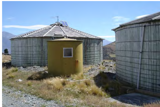
Photo 2: Reservoirs and chlorination shed
