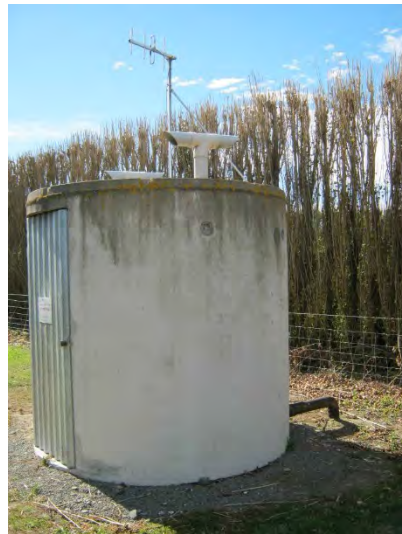
Photo 2: Otahuna Valley pump shed
