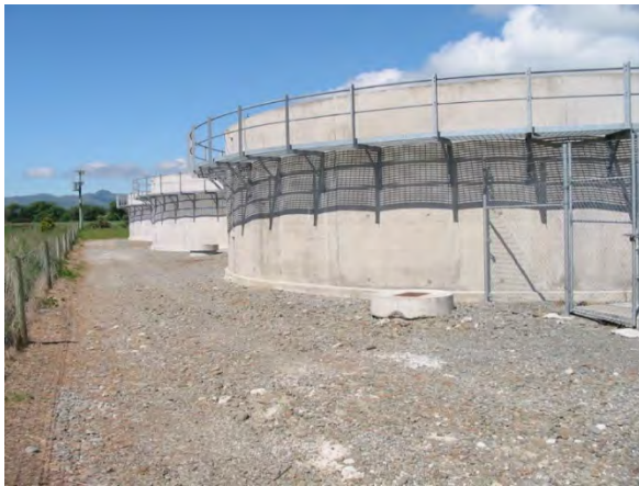
Photo 1 – Buffer storage tanks
