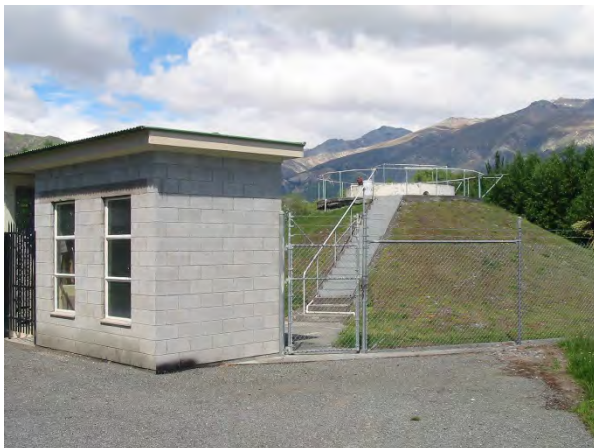
Photo 1 – Pump house and Imhoff tank
