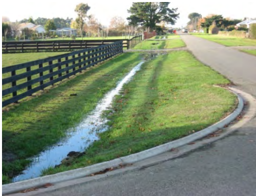
Photo 1: Typical swale after light rain
