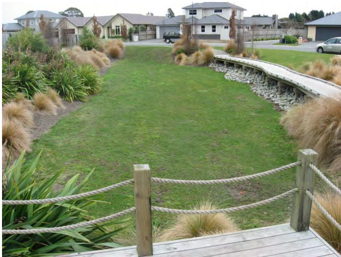
Photo 1: Typical Stormwater Infiltration Basin
