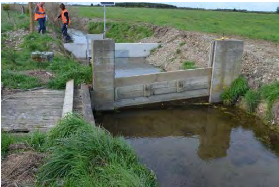
Photo 3: Typical flow gauging site
