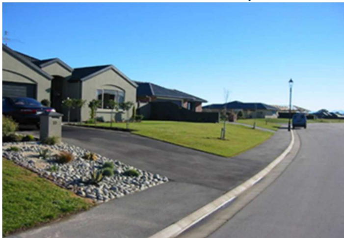
Figure 9.1.2: Low Profile Kerb and Channel and Entranceway
