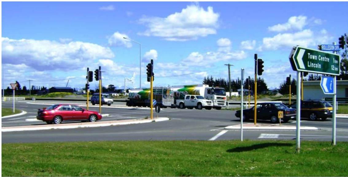
Figure 7-18: New Traffic Lights at Rolleston and State Highway 1 (partially paid by Developer Contributions)
