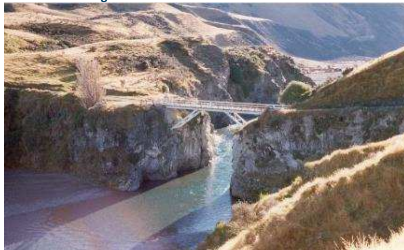
Figure 9.1.8: Poulter River Bridge – Mt White Road
