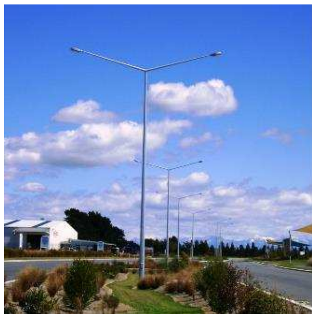
Figure 9.1.4: Double Arm Street Lights, Izone Drive
