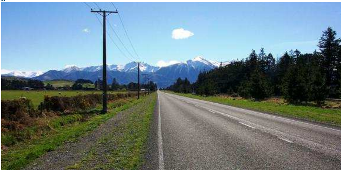
Figure 9.1.1: Rural Sealed Pavement and Shoulder
